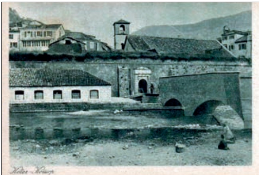
Sl. 9 | Kameni most sa puškarnicama i pokretni drveni most s kraja XIX vijeka (Iuri Gagarin, Medieval entrance with drawbridge with chains and iron grating on stone wall)
